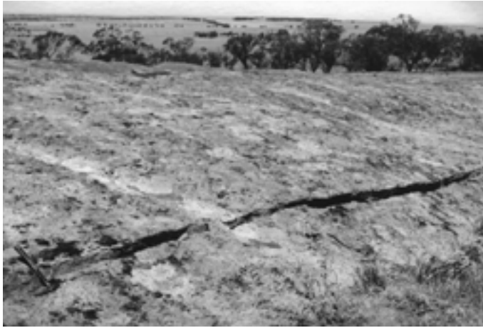
Figure 10. Fault developed in the late morning of 19 January, 1999, on Minnipa Hill, northwestern Eyre Peninsula, South Australia.
