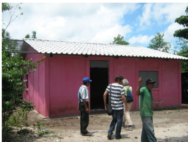
Exterior vivanda rematada (vense as correas sen cortar)
