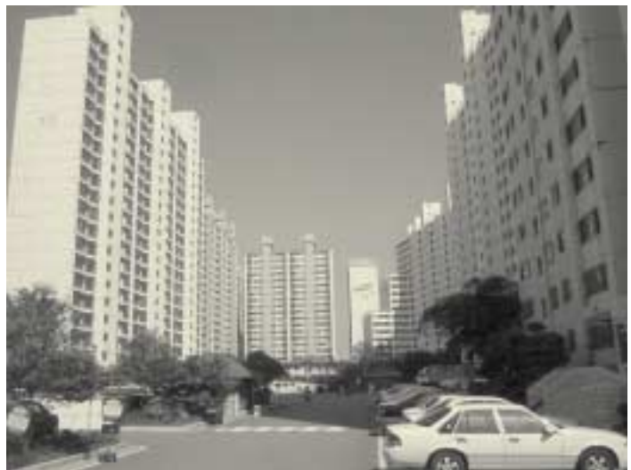
Figure One: Typical Apartment Buildings in Daegu, South Korea.
